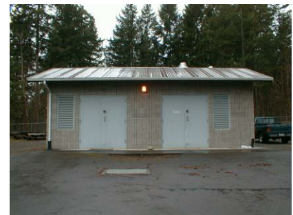
Tacoma Point Well No. 2 Building
