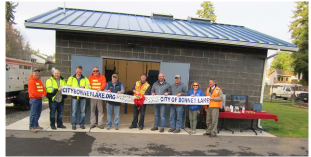
84 th Street Booster Pump Station
