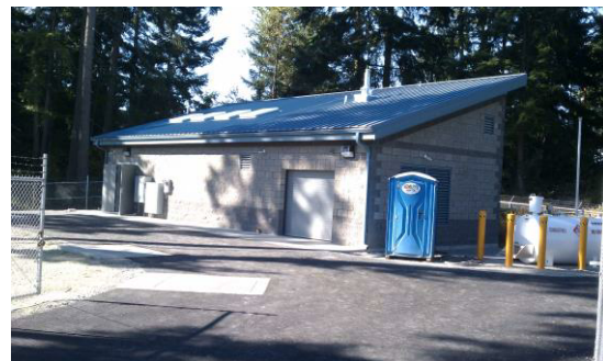
Prairie Ridge Booster Pump Station
