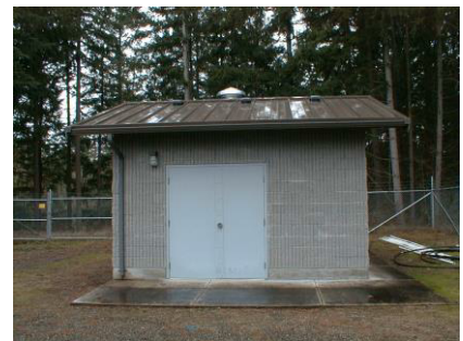
Tacoma Point Well No. 4 Building
