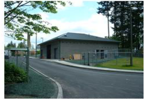
Ball Park Well No. 2 and Treatment Facility
