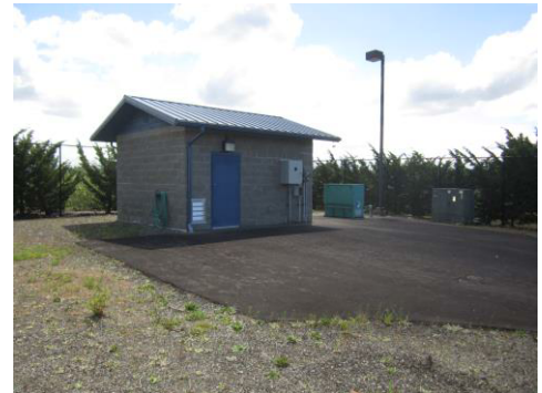
Panorama Heights Booster Pump Station
