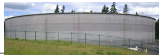
Peaking Storage Reservoir
