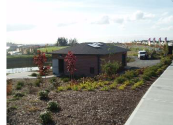
Pinnacle Estates Booster Pump Station
