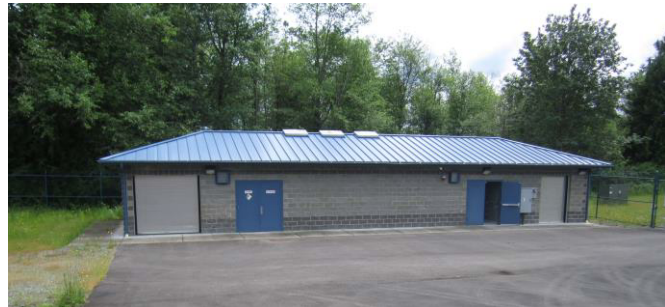
Peaking Storage Booster Pump Station
